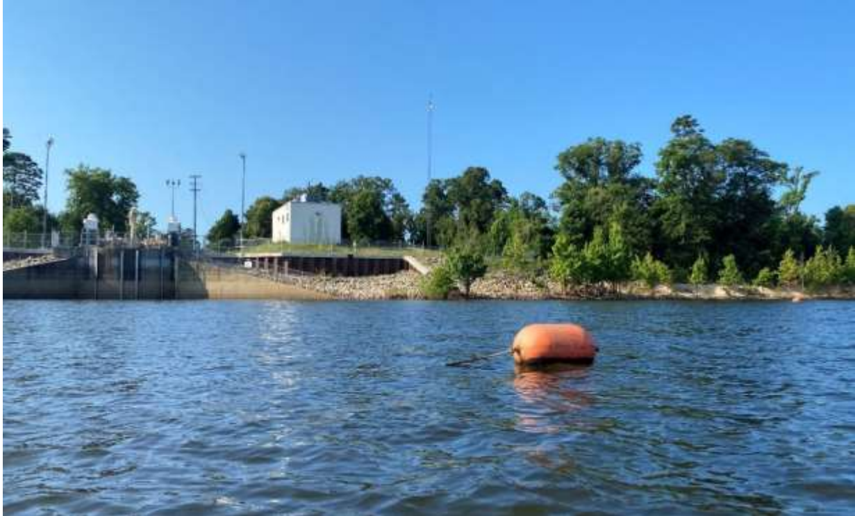
Figure 35: City of Longview Intake
